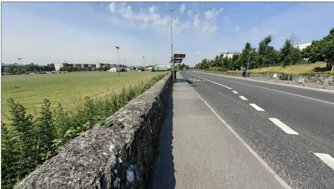
Plate 15.33: View WNW along south side of Dublin Road between Skerritt Roundabout and Ballyloughan Road (opposite ATU Galway City). Designs include the removal of this modern wall and a thin sliver along the edge of the playing pitch
