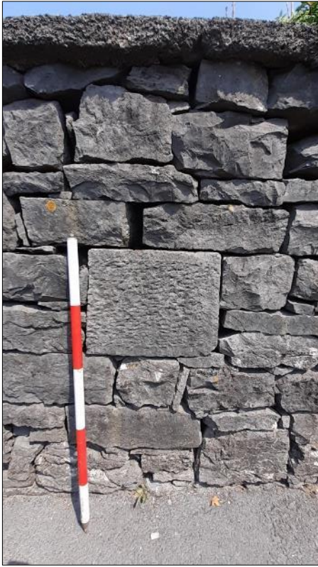
Plate 15.24: Closeup of punch-dressed stones (CH006) showing ashlar construction
