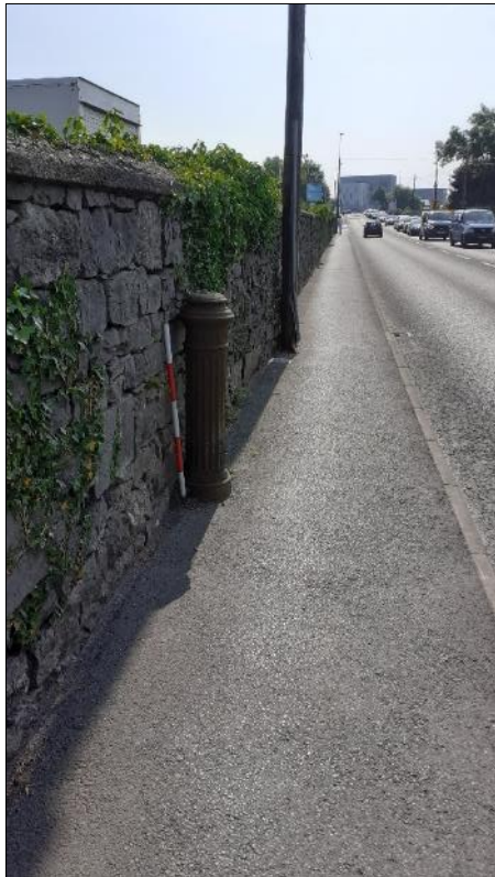
Plate 15.20: Vent pipe (CH007), facing ESE
