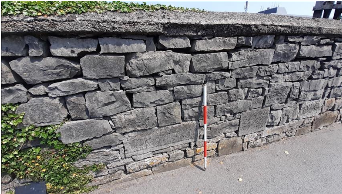
Plate 15.22: Boundary to Galwegians RFC (CH006) facing north. Showing punch-dressed stones amongst the roughly hewn blocks
