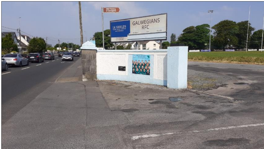
Plate 15.26: Entrance to Galwegians RFC, showing memorial plaque (CH008), facing WNW. The roughcast rendered wall of the entrance appears modern
