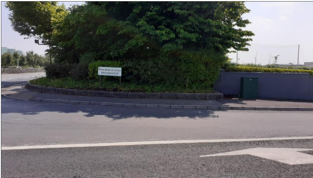
Plate 15.31: Junction of Ballyloughan Road, facing ESE showing low stone kerb and green area to be removed. The kerb contains cut stone but none appear to contain medieval fabric
