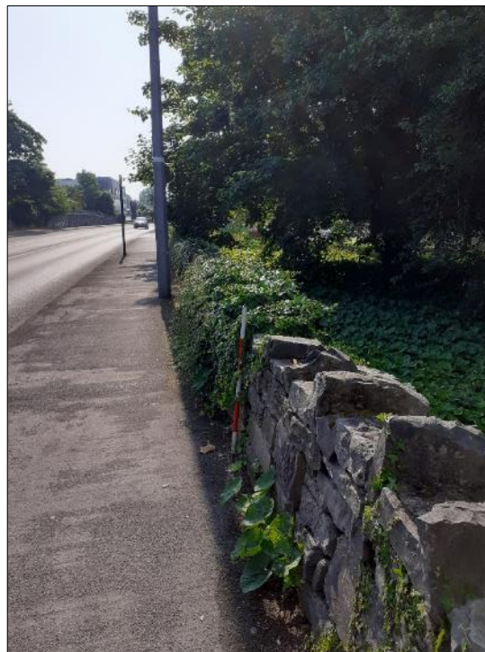
Plate 15.3: Modern wall and green area along south side of Dublin Road, facing ESE. The wall and part of the green area to be removed
