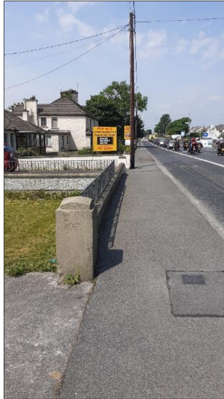
Plate 15.17: Existing footpath on south (to be side of Dublin Road, facing WNW
