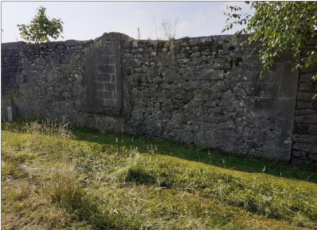
Plate 15.10: CH003, facing south showing ashlar quins and window surrounds
