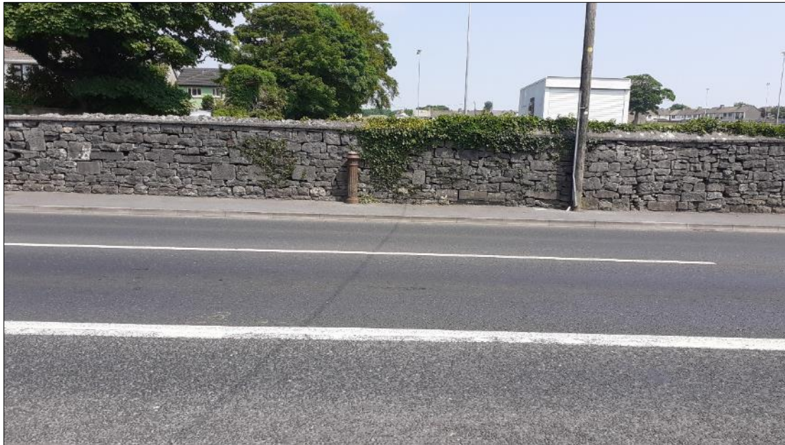
Plate 15.19: Boundary to Galwegians Rugby Football Club (RFC) (along north side of Dublin Road), facing north. The wall (CH006) and vent pipe (CH007) are not designated cultural heritage features. The wall is of semi-dry stone construction, containing roughly hewn blocks and re-used punch-dressed limestone built to courses and topped with concrete coping. This may be the boundary to Glenina House (also the townland boundary between Ballybaan Beg to the north and Rinmore) as depicted on the 25-inch OS map (c.1900) or may be a re-build on the same alignment
