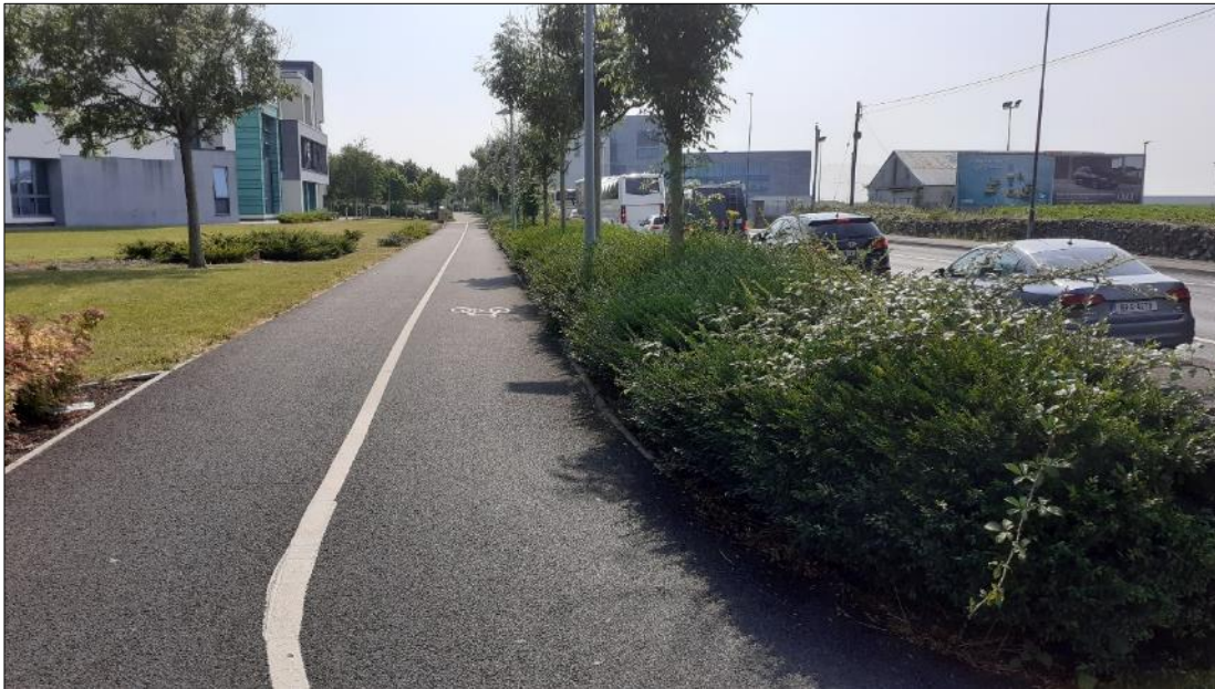
Plate 15.32: Existing cycle lane and footpath within ATU Galway City on north side of Dublin Road, facing east towards Skerritt Roundabout
