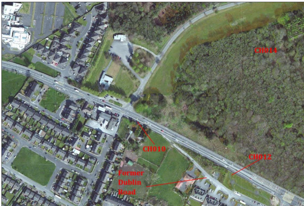
Figure 15.18: Aerial view showing the entrance to Merlinpark demesne CH014, the location of cut stone CH010 and vent pipe CH012.
