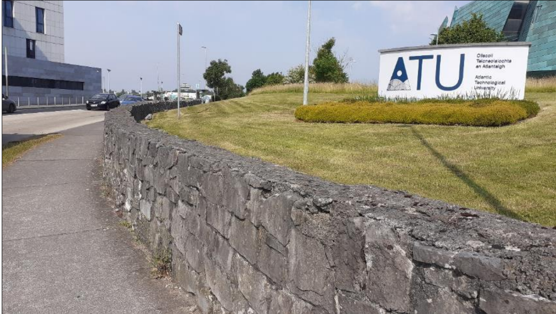
Plate 15.34: Modern retaining wall of ATU Galway City from Skerritt Roundabout, facing west
