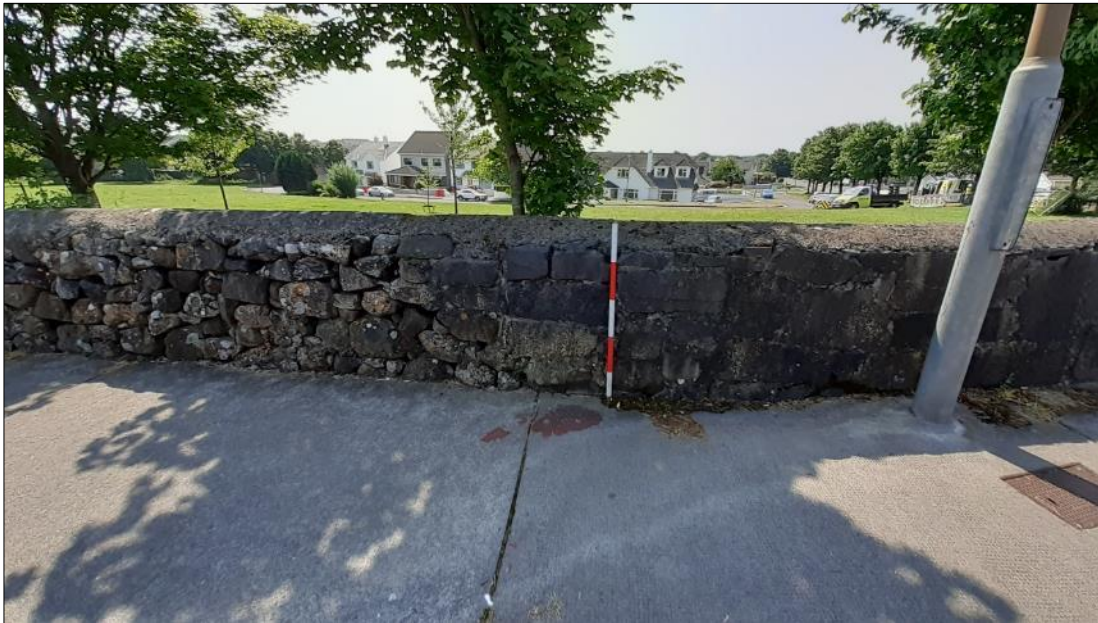
Plate 15.36: Wall along south side of Dublin Road immediately east of Gleann Rua. Note the composite construction of the wall, which will be partially removed as part of the design. The wall appears to be modern and not the same wall as depicted on historic OS maps
