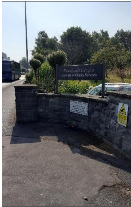
Plate 15.5: Modern entrance and wall to Brothers of Charity to be removed along south side of Dublin Road, facing ESE
