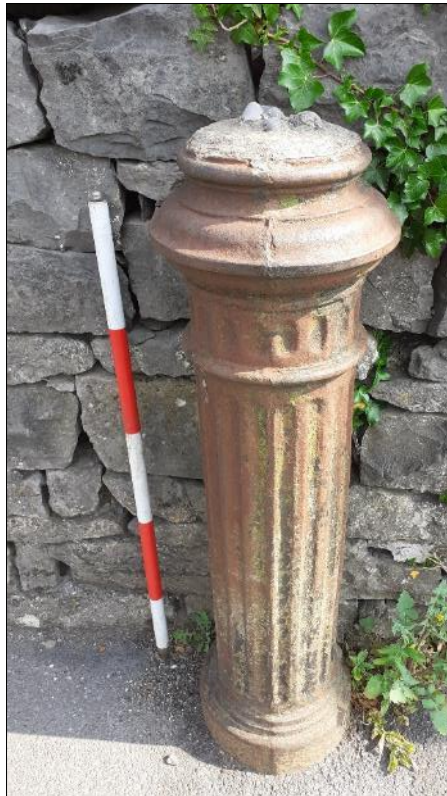
Plate 15.21: Vent pipe (CH007), facing north
